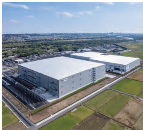
The newly established Sarugashima Center (opened in February 2025) serves as a hybrid distribution center, delivering both dry and chilled products simultaneously.
